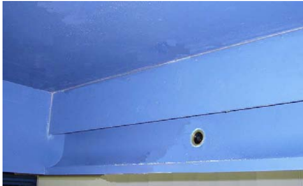
Figure 7: Air inlet section and the position of upstream camera.
