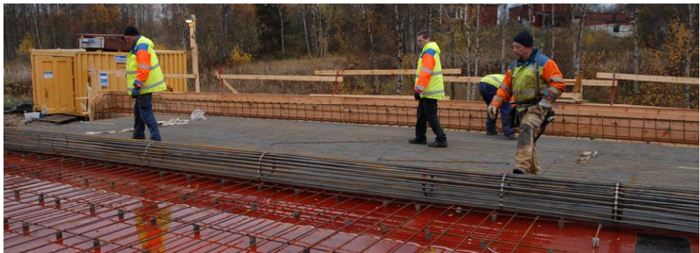
Figure 12: Rebar carpets, rolled out on the superstructure at the Kalix project.
