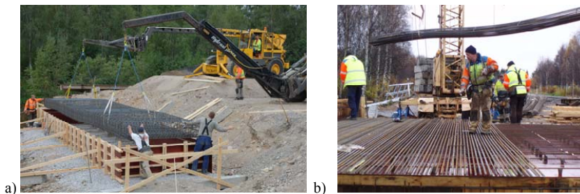
Figure 3: a) Placing prefabricated reinforcement for a foundation. b) Reinforcement carpet lifted into place.
