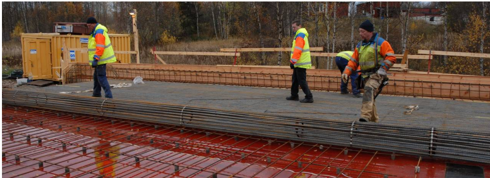
Figure 11. Rebar carpets, rolled out on a superstructure at a studied project.
