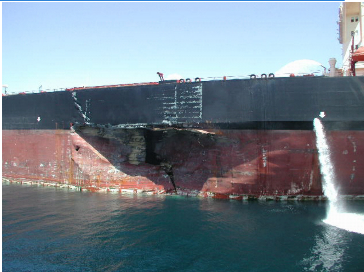
Figure 3 A VLCC after a collision with an OBO in ballast. The collision angle was about 90 degrees. The penetration is about to B/5.
