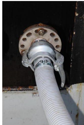
Picture 4. Connection of sludge hose on board.
