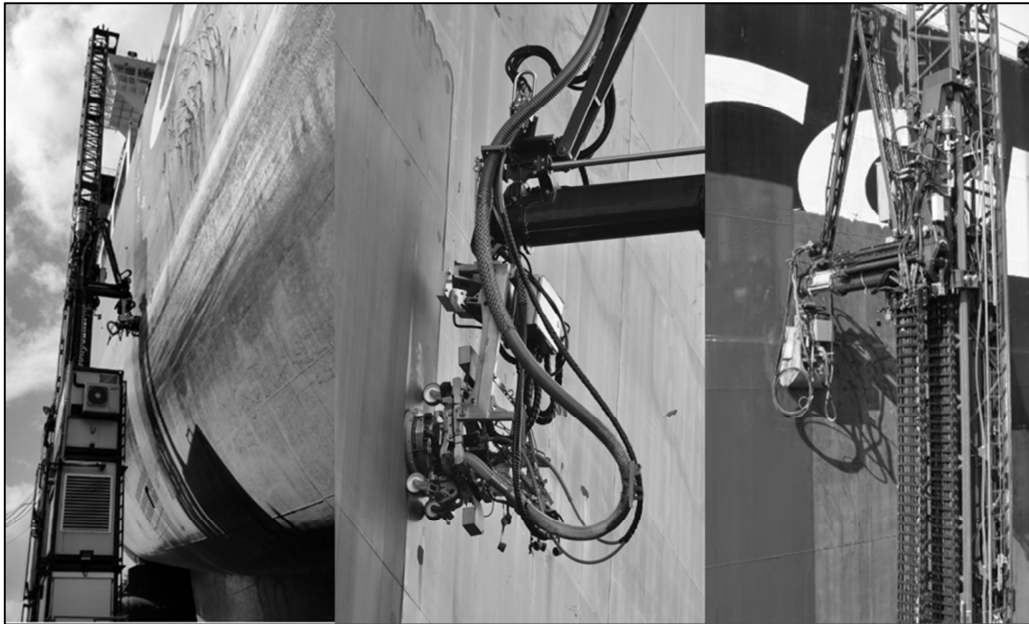
Fig. 1: Automated Hull Treatment Carriere (HTC), left to right: washing, ultra-high pressure water jetting, recoating
