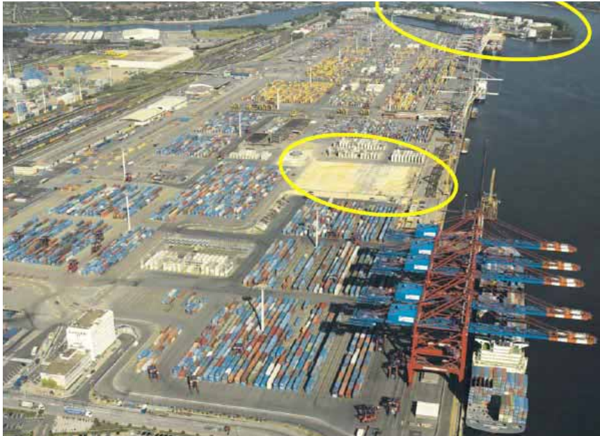
Figure 65: Eurogate Container Terminal Hamburg
