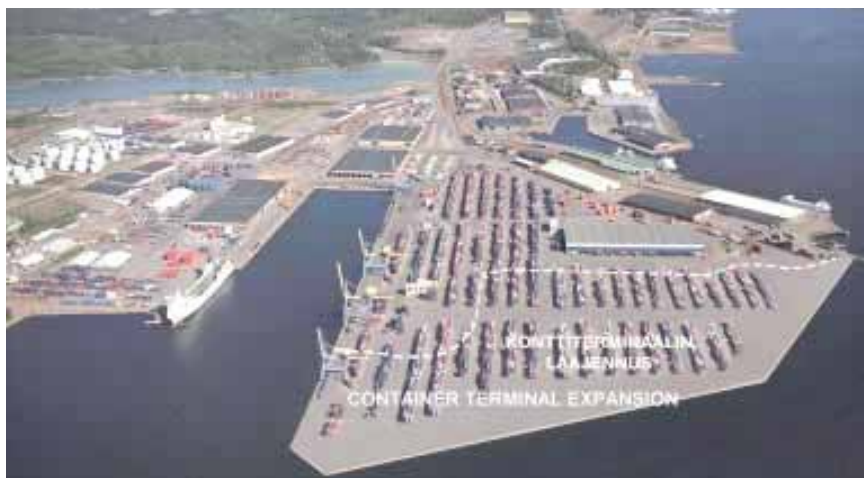
Figure 47: Port of Hamina container terminal extension
